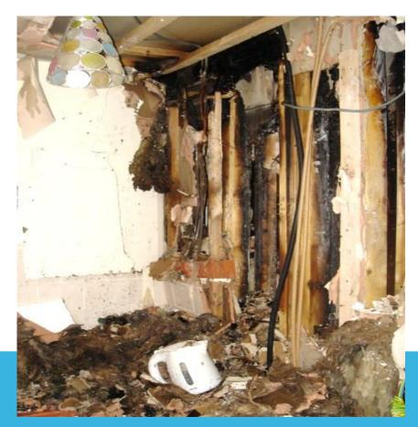
Fire Spread in Wall Cavities between Apartments.
